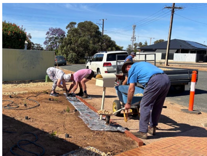
Landscaping works at Bagshaw House
