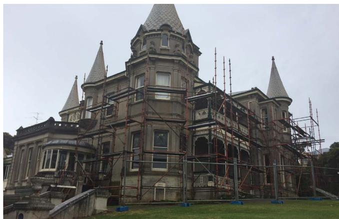
The project is reasonably complicated due to the height and design of the building. Scaffolding surrounds the building to provide a safe working environment for the tradespeople involved in the project. In addition to replacing the roof cladding and gutters, all of the fascia boards and scotias will either be repaired or replaced as well as painted and a damaged chimney will be repaired.
